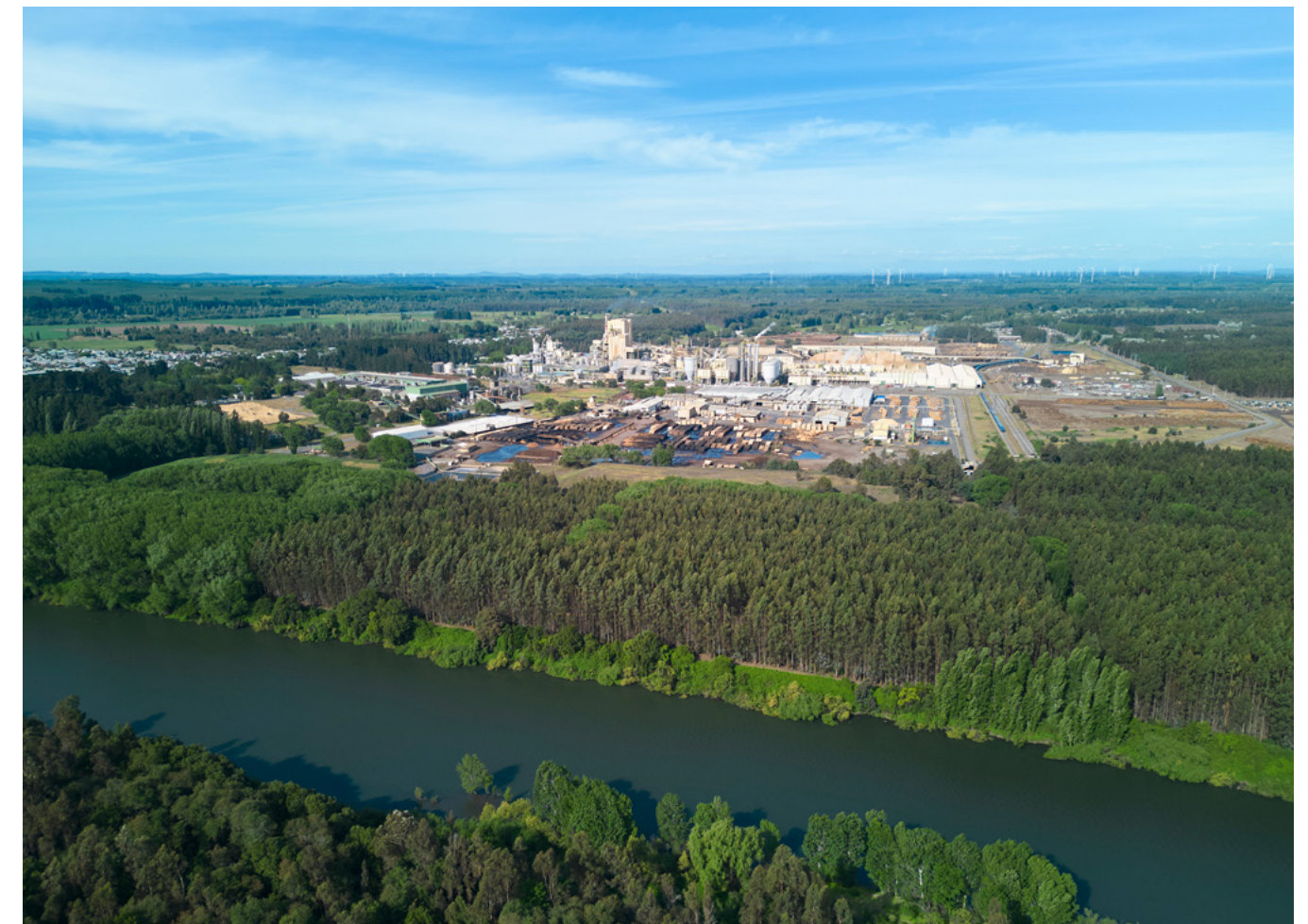
Santa Fe Plant, Chile.
