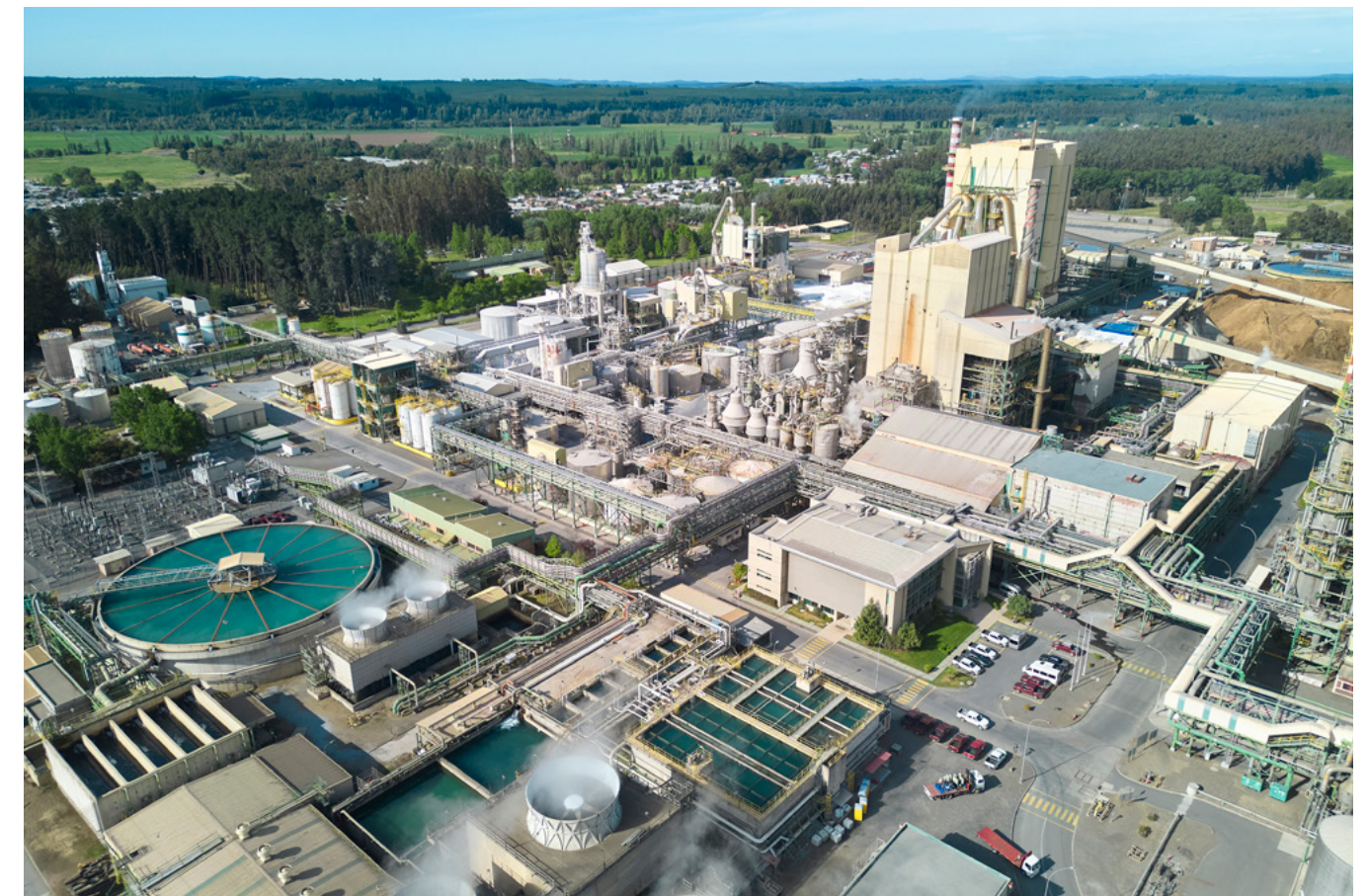
Santa Fe Plant, Chile.
