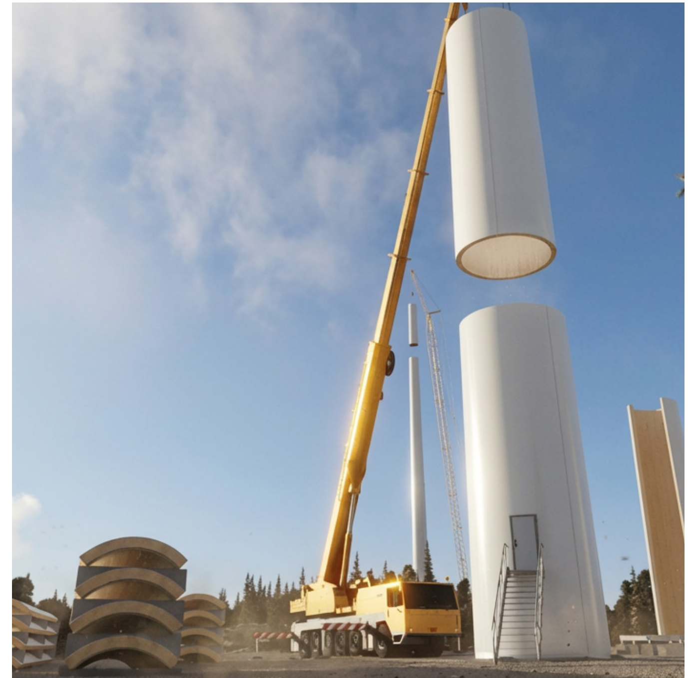
Wooden wind turbine tower assembly developed by Modvion.
